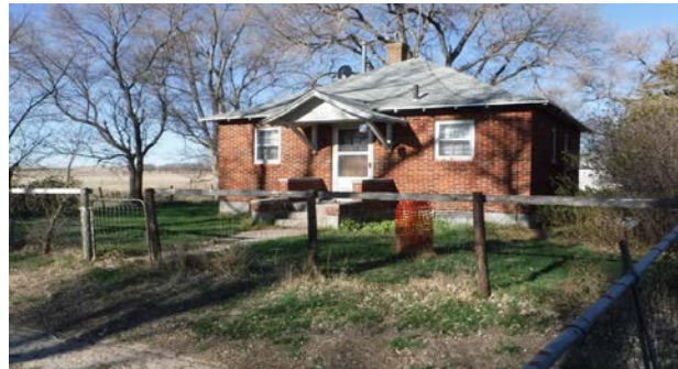
Brick House at LO00-001, view west-southwest
