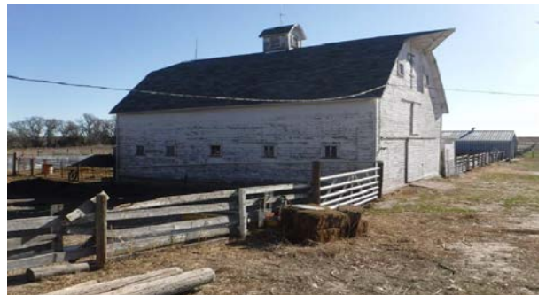
Barn at LO00-001, view northeast
