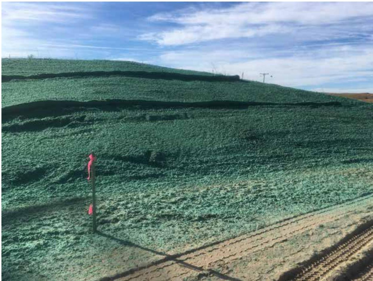
As part of its work to stabilize sites, NPPD applied stock-piled topsoil, drilled a native seed mix, installed straw wattles, and applied hydromulch to the expanded Thedford substation.
