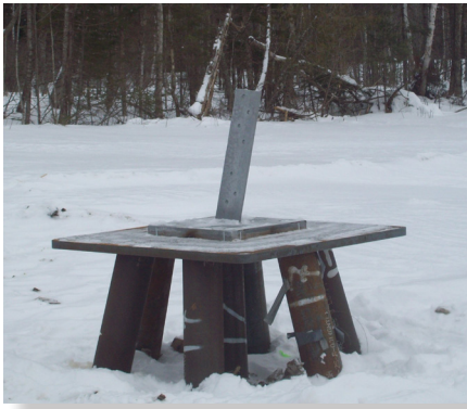
The helical pier foundation shown above is for a 500 kV self-supporting structure and is therefore larger than what is expected for a typical R-Project foundation.
