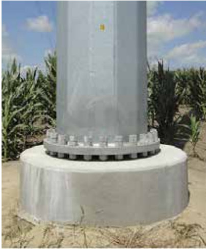
Drilled Pier Foundations. Materials: Concrete, Steel Rebar, Anchor Bolts / Stub Angle Equipment: Digger, Concrete and Dump trucks, Crane
