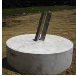
Drilled Pier Foundations. Materials: Concrete, Steel Rebar, Anchor Bolts / Stub Angle Equipment: Digger, Concrete and Dump trucks, Crane
